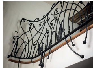
Organic balustrade: Constructed using forged and fabricated techniques and finished in bees' wax
